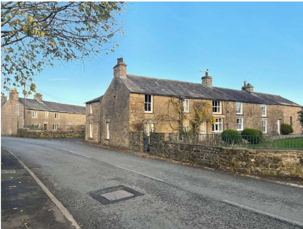
Figure 25: Main Street looking north with sandstone farmhouses built perpendicular to the road
