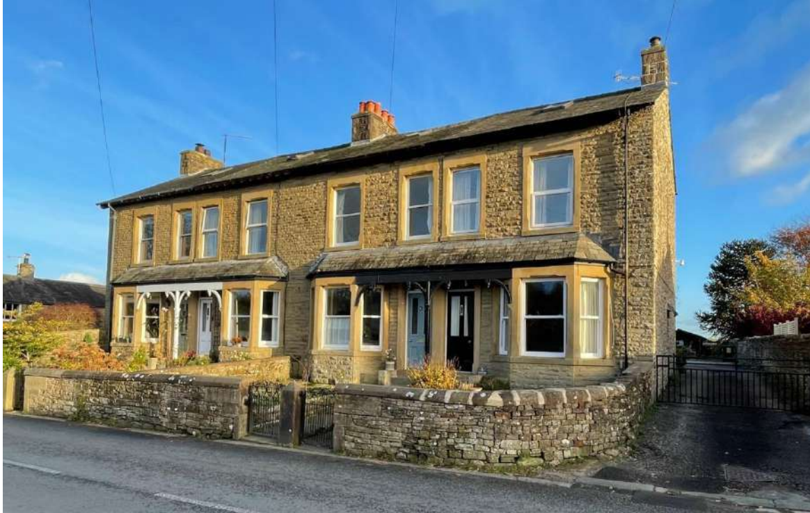
Figure 31: The Chestnuts (previously The Villas), Main Street
