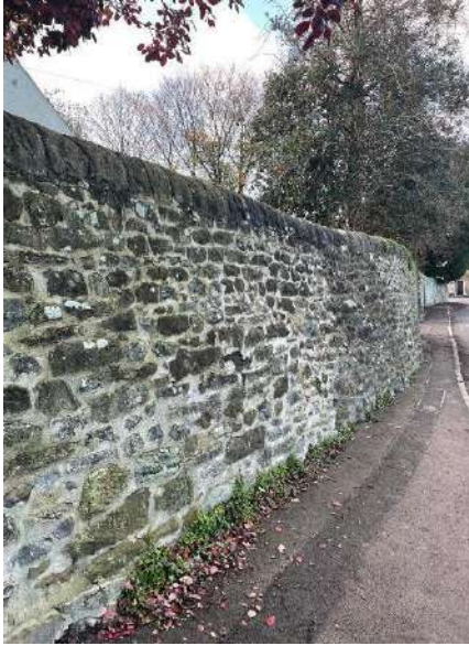
Figure 52: Hogsback topped wall leading from Main Street to Church Street
